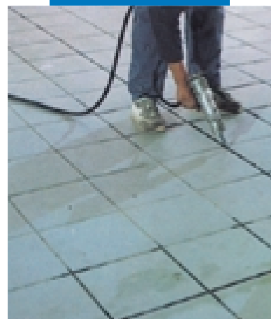
Sealing ceramic tile floor with Mapesil AC
