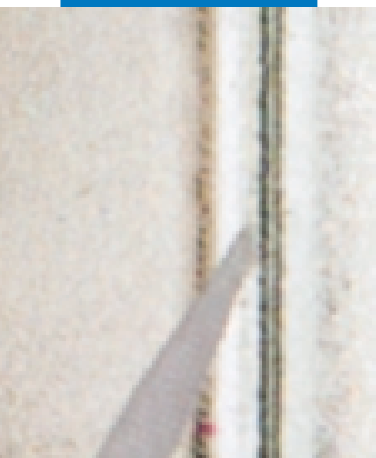
Sealing U profiled glass
